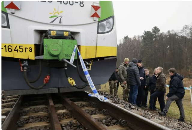
Polish Prime Minister Donald Tusk, second right, visits the site of the railway track that was damaged near Deblin, Poland. (KPRM/AP)
